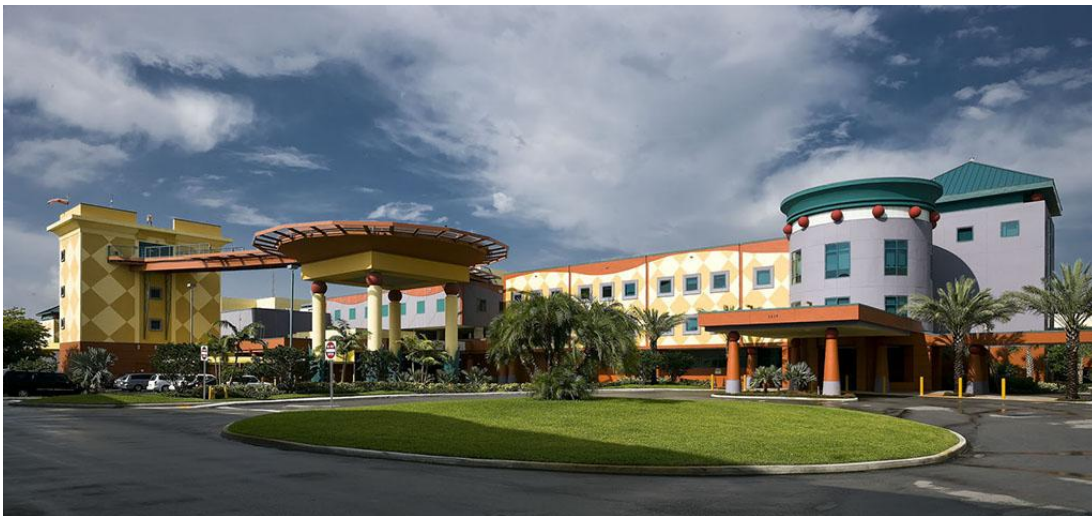
Figure 6: Nicklaus Children's Hospital following 2001 retrofit [29]
